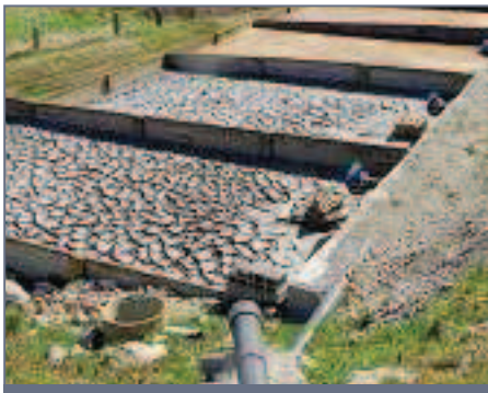
Polymer dry stacking, showing two stages in the precipitation of solids from contaminated sediment
